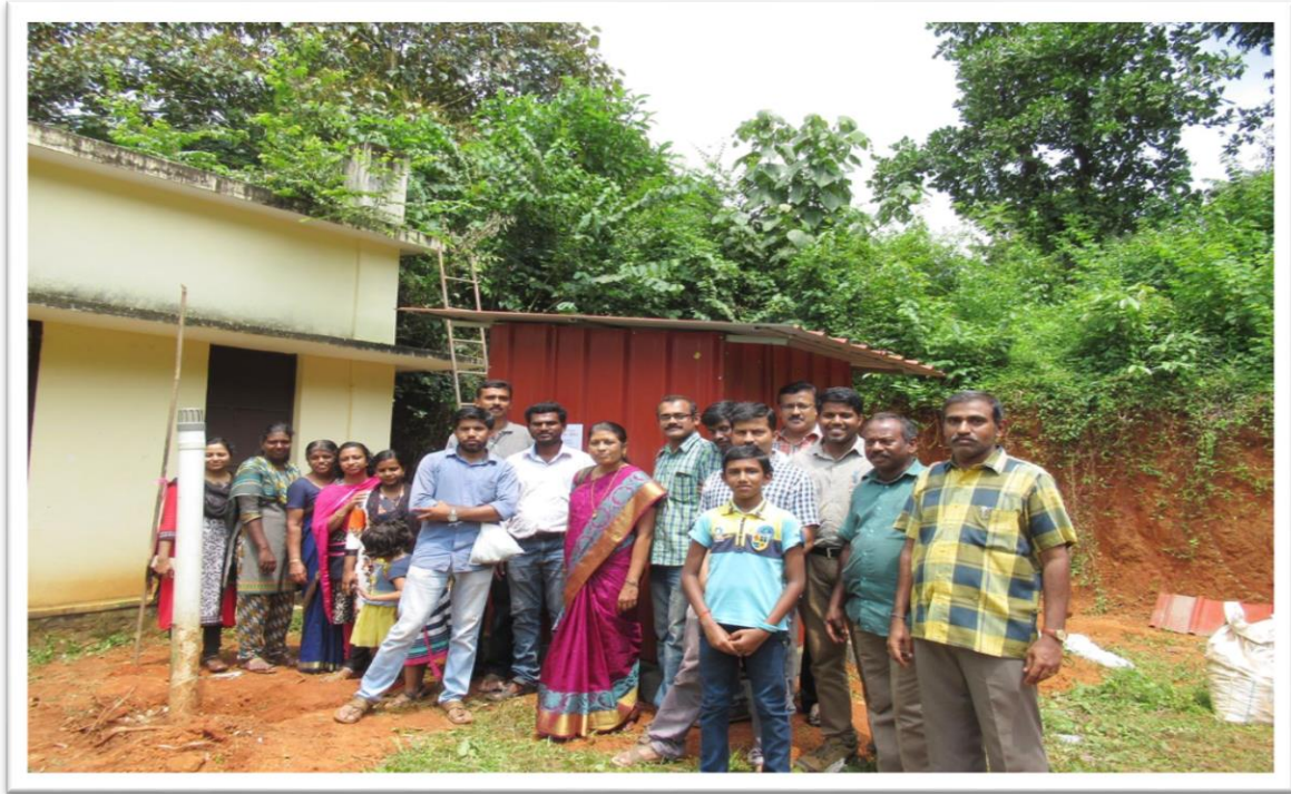
Newly constructed toilet facility for Harijan Colony, Chakittapara panchayat, Calicut
