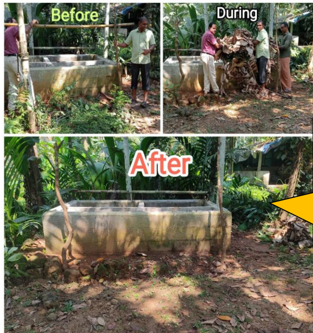
View of vermicompost unit rebuilt at Maruthonkara, Kozhikode
